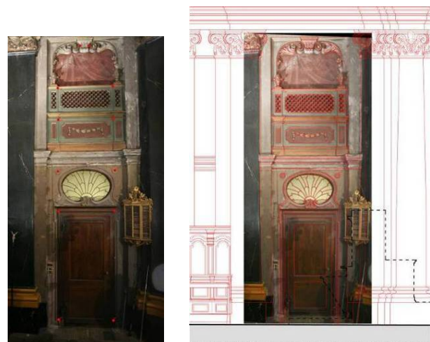
Figure 8: Original photo and rectified photo employed for the representation of the decorative elements for the section representation
